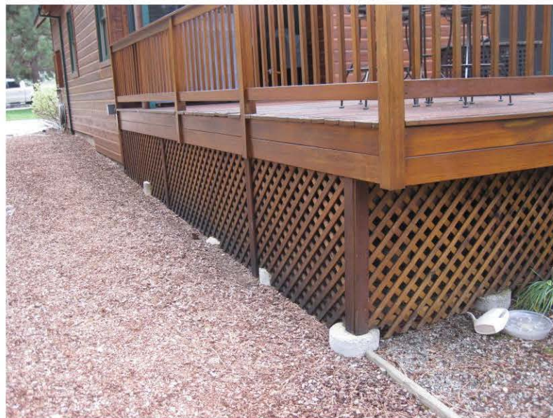
Photo 10-Lattice beneath a deck
