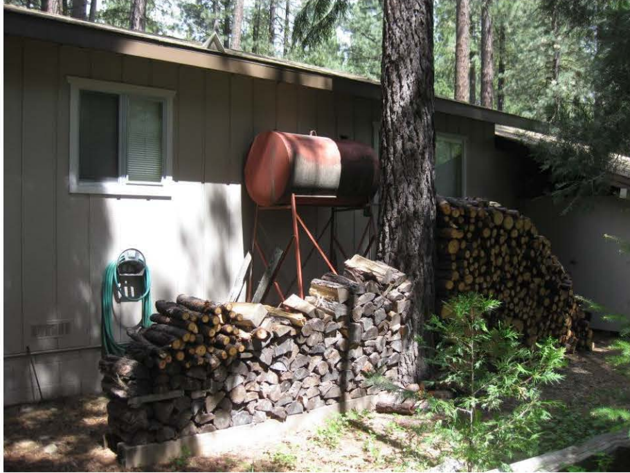
Photo 16-Firewood should not be stored near fuel tanks
