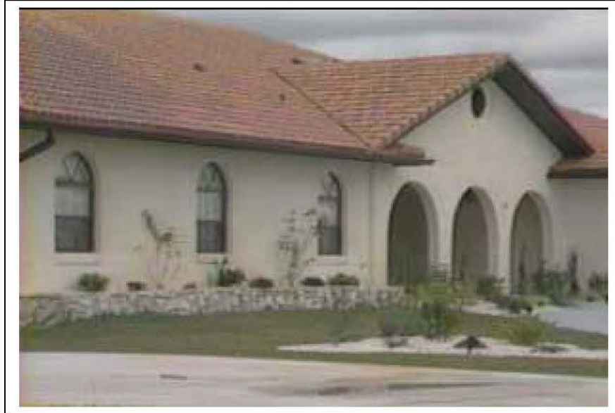
Photograph 11.3. Noncombustible Roof
