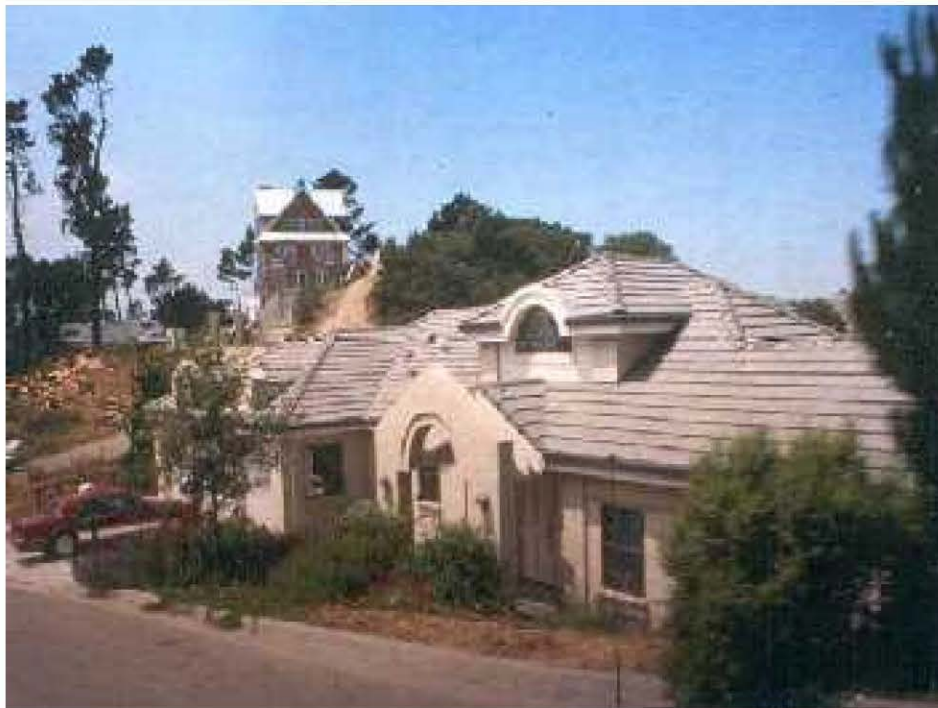
Photograph 11.1. A Clean, Well-Maintained Class A Roof
