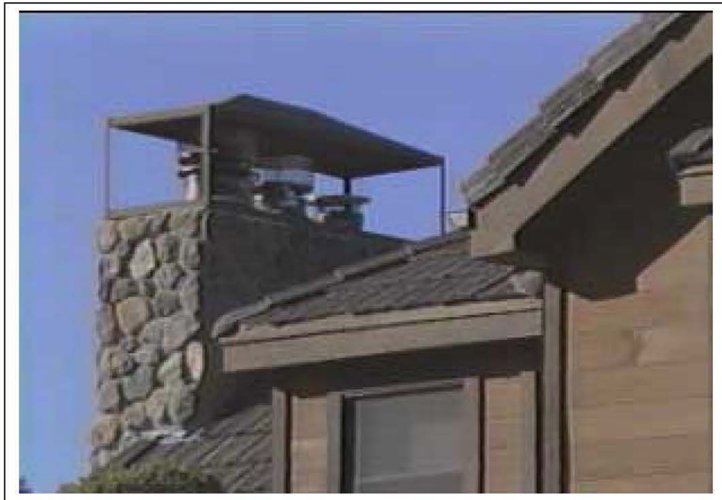
Photograph 11.2. Chimney/Stovepipes with Spark Arresters
