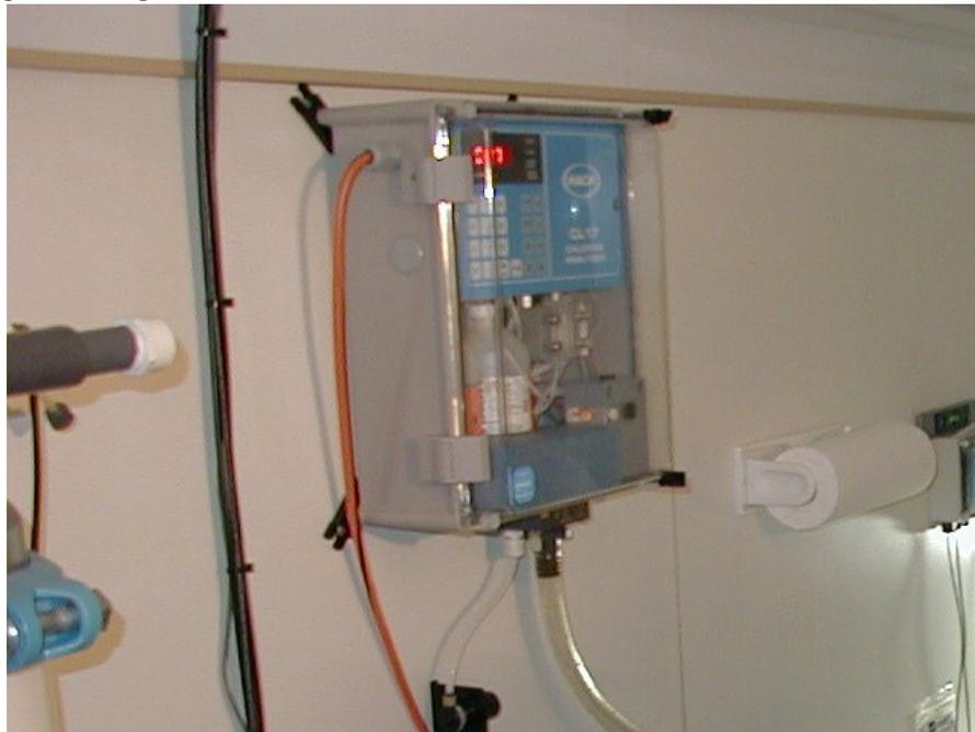
The front one-half of the trailer is shown above. The instrument foreground on the wall is an in-line chlorine analyzer. The smaller boxes on the wall above the light are electronic flow meters used to monitor cumulative as well as instantaneous flow for each treatment train in the pilot plant.
